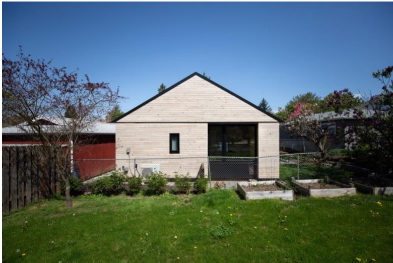
The space between Scott and Lauren's ADU and the existing bungalow, which they rent out to tenants, functions as a communal yard and garden. (Photo by Lucy Wang)
